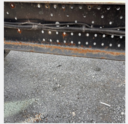
Acceptable corrosion for age
